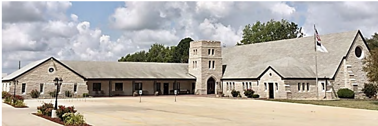
Current HCC building on North Vine Street (old Route 51)
